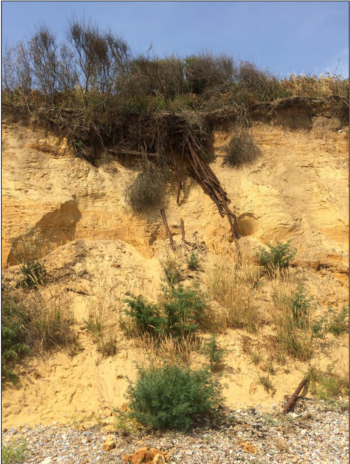
Plate 1: Traces of coastal defences eroding from clifftop at Thorpeness
